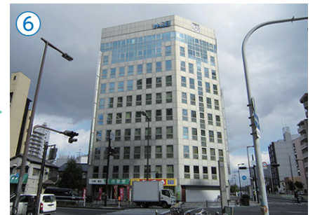
6 Nichidai Wasei Building.
