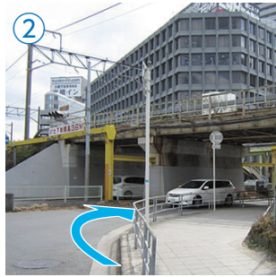
2 Go under the elevated structure.
