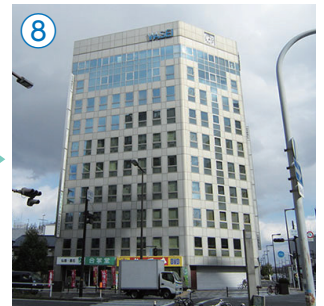
8 Nichidai Wasei Building
